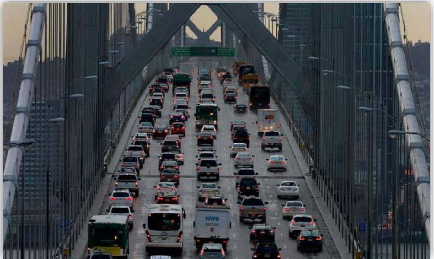
San Francisco-Oakland Bay bridge.
